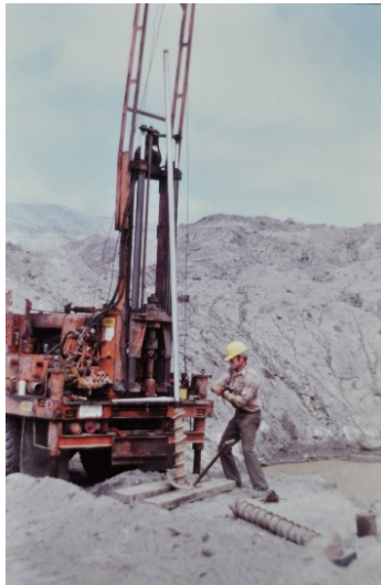
Ron Lane installing piezometers in Coldwater Lake blockage—unstable natural dam impounding the lake. (Photo by K. Tanner, July 1981).
