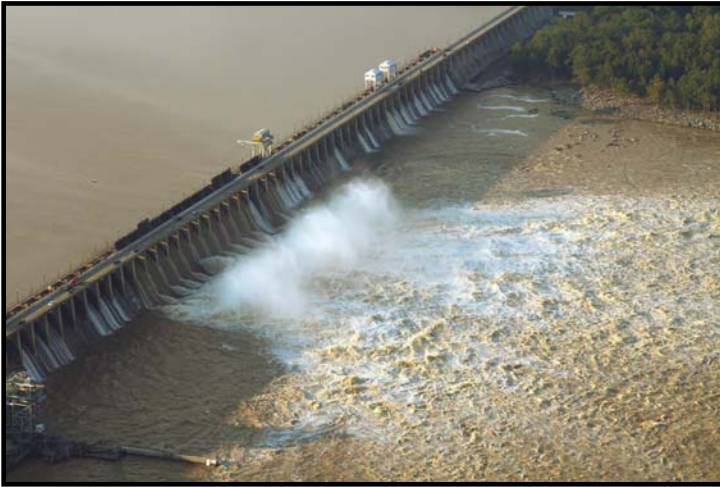
View of the Conowingo Dam on the Susquehanna River in the aftermath of Tropical Storm Lee. Discharge at time of the photo was 220,000 cubic feet per second (cfs). Peak discharge for the flood was 778,000 cfs.
